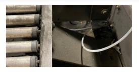
A customer wanted to eliminate the hassle of brushing oil onto chains. The goal was to reduce the amount of manpower needed to lubricate the machine. GreasePoint and the PennAir Field Service teams installed the system before the next plant production run. The installation will help improve component life, machine accuracy, safety, production, lube efficiency, and reduce waste.
